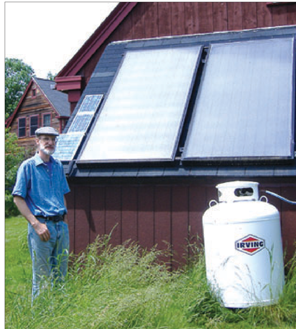
Guy Marsden and his Solar Collector
